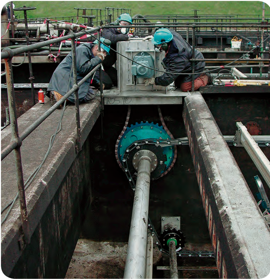
API sedimentation tank in the refinery
