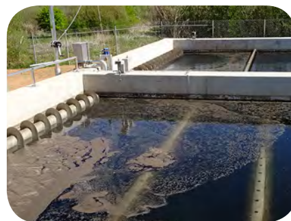
Rectangular tanks with submerged drain tubes and screw conveyors for floating scum removal
