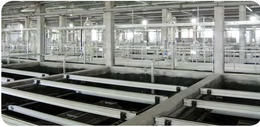
DAF-scrapers totally made in plastic
