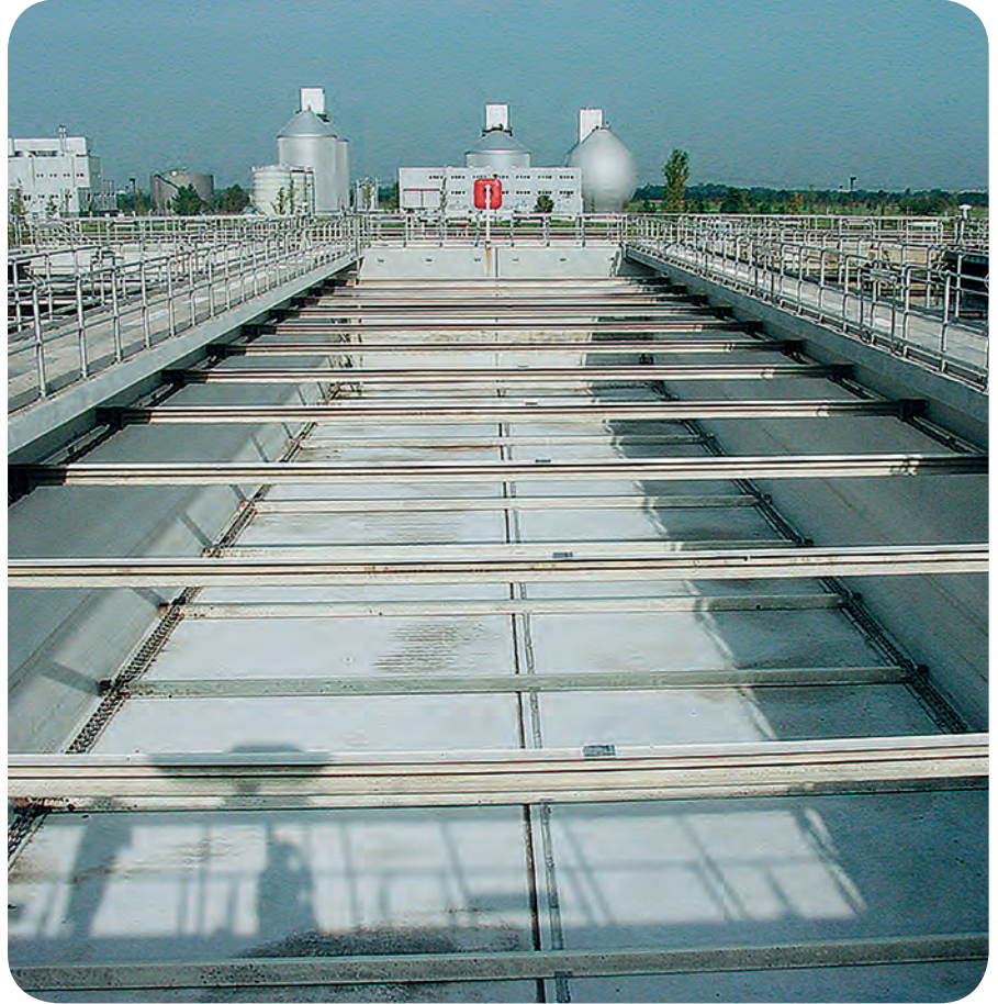
Bottom sludge and floating scum scrapers
