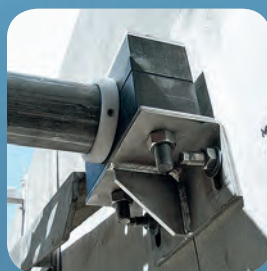
Partitioned bearing supports
