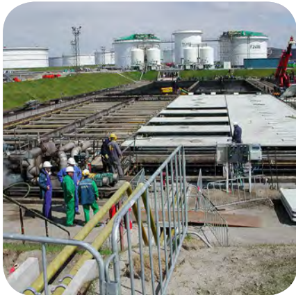
Refinery, the Netherlands
