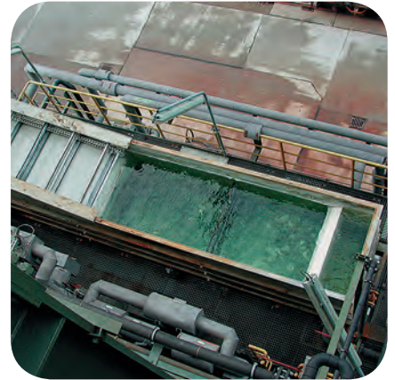
Flotation plant made entirely of non-metallic materials
