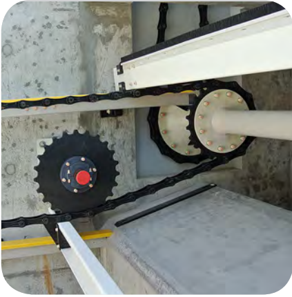
Flotation scraper made entirely of synthetic materials
