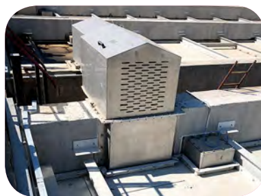
API tanks, gas-tight
