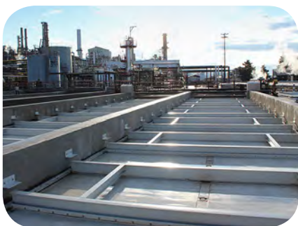
API tanks with floating covers
