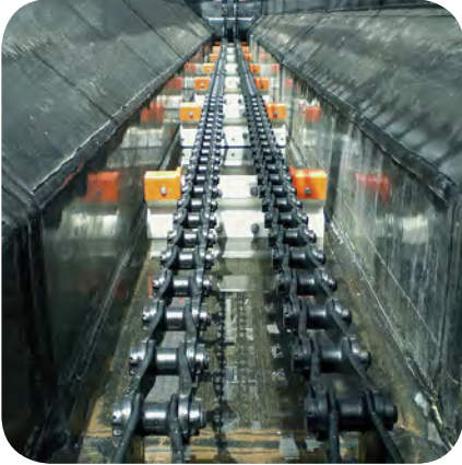
Grit collector scrapers
